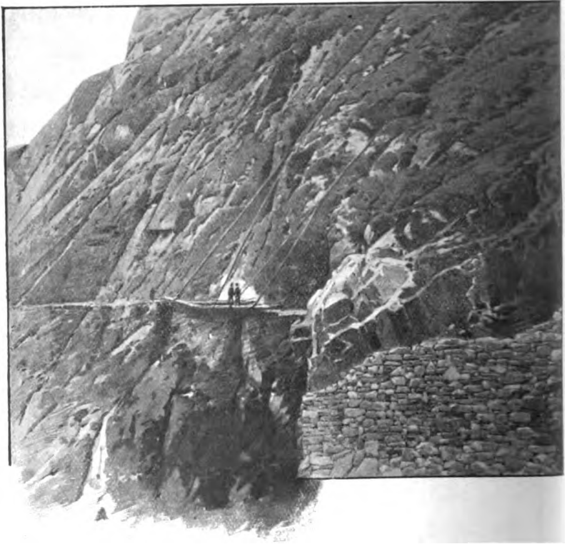
A SHAKY PASSAGE ON THE NERPANI ROAD
